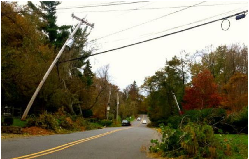
Figure 2: Wind Damage from Hurricane Sandy Source: Rumson-Fair Haven Patch
