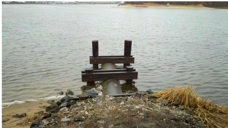
Figure 5: Waterman Avenue Stormwater Outfall
