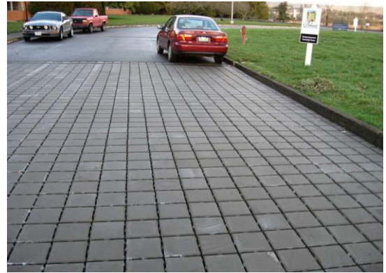
Figure 10: Permeable Pavements (Source: EPA)
